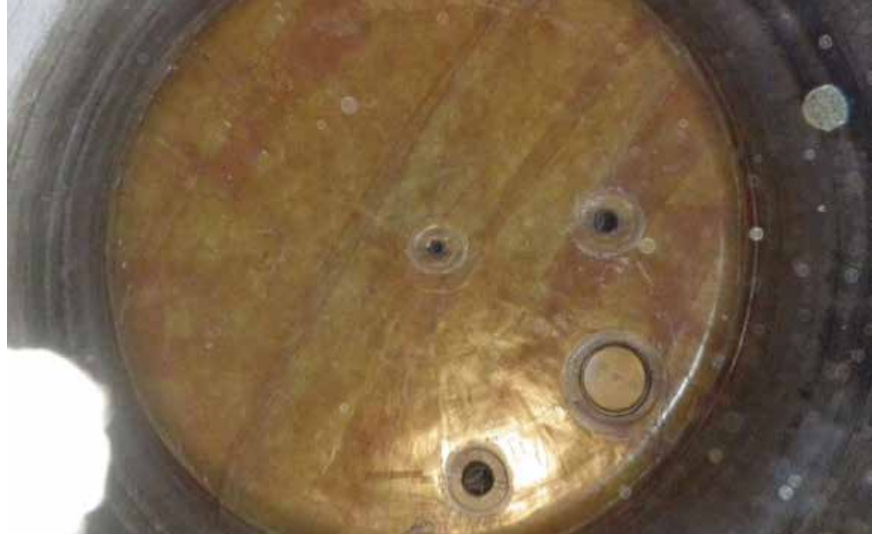
THE PHOTO OF THE ROOF OF THE TANK.
